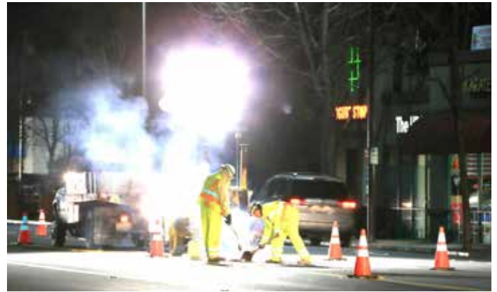
Fig. 5 - High-Level Gain: Darker areas are seen better than before, but bright spots are clipped and detail is lost.
